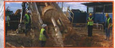
Horizontal directional drilling / Reamer
